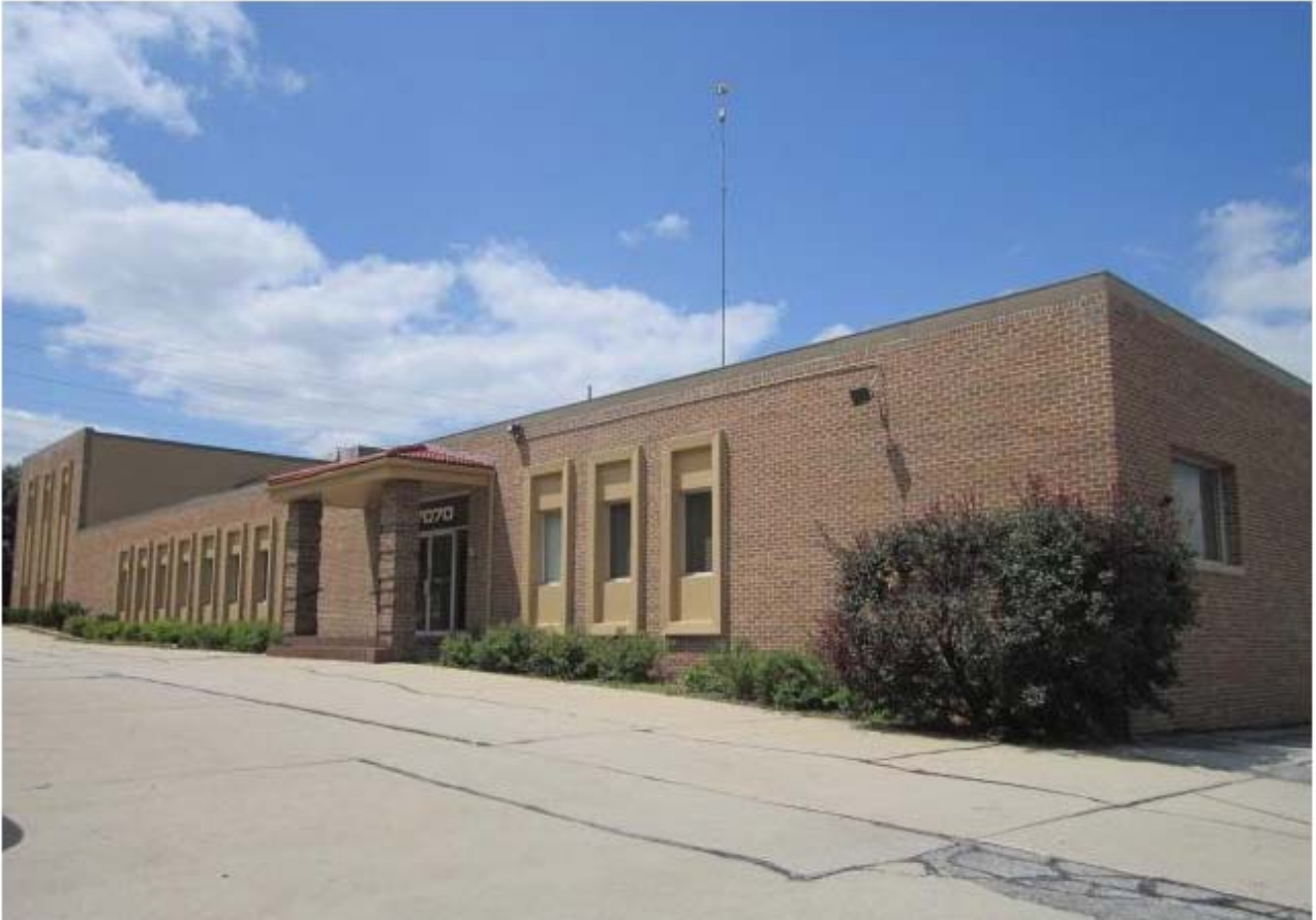
View from the Southeast
